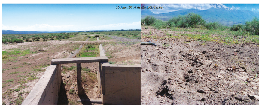
Figure 2. Severe wind erosion, sediments filled the irrigation channel in Aralik-Igdir/Turkey.
