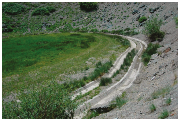
Figure 1. Mine spoil mitigation after installing soil cap that is protected from further contamination by stormwater runoff using collection and diversion channels.
